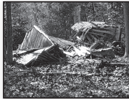
Collapsed cabin on Sepous Road property
