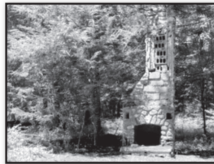
Fireplace remaining on Sepous Road property
