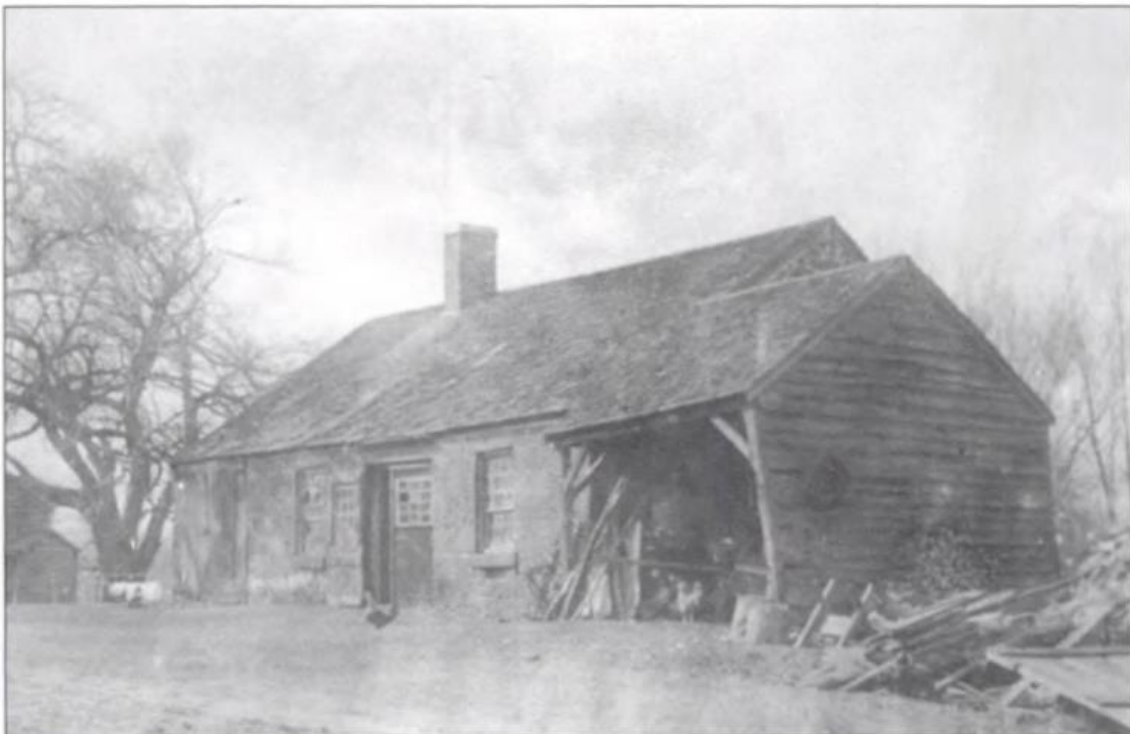
"NORTH'S BLACKSMITH SHOP, 1911." Built in 1832 by Joseph North, this building still stands as the Forge Room of the Avon Old Farms Inn. Blacksmiths made shoes for horses and oxen, repaired and sharpened farm implements, put iron on wagon wheels, and did other work. (Clinton Hadsell photograph, Avon Collection, courtesy of Doris Miller.)
